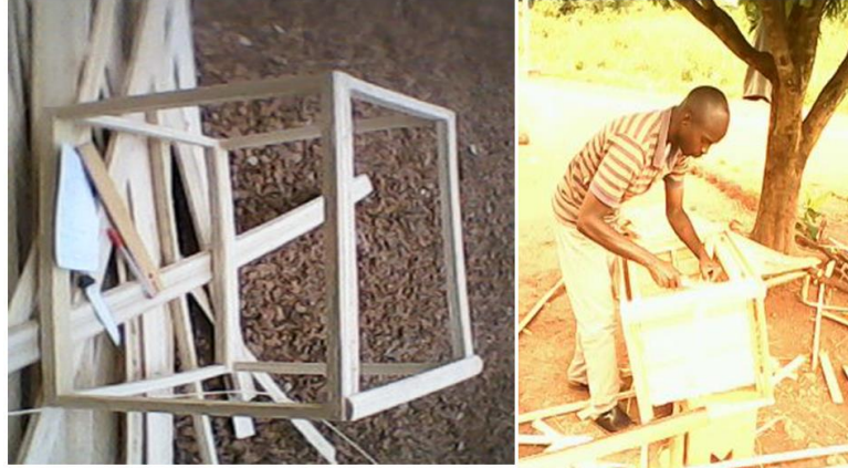
Figure 1. Part of the Inner Wall and Internal Wall
