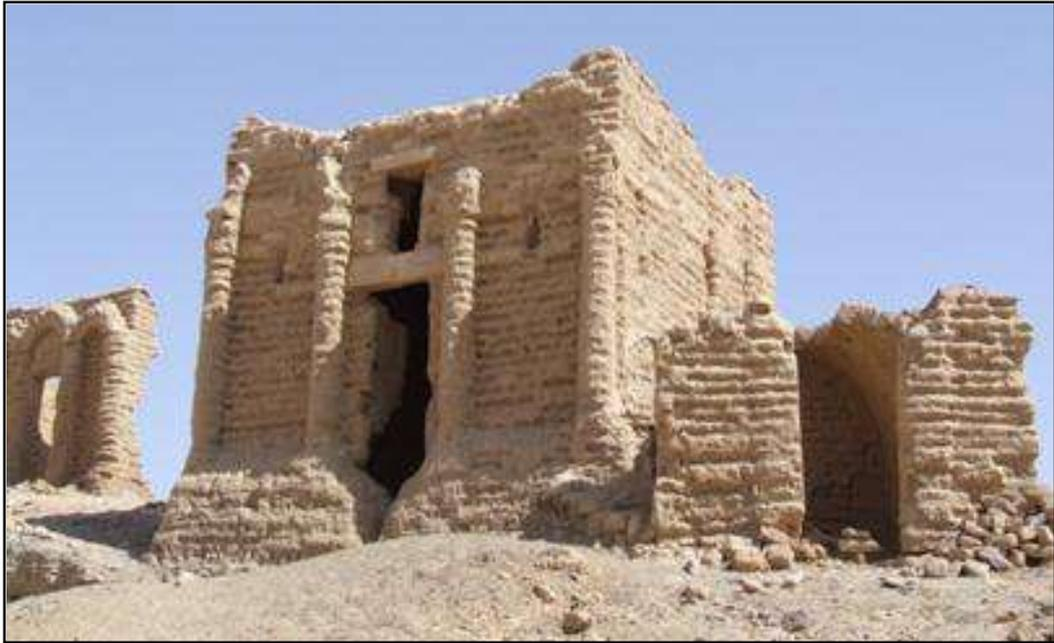
**Figure 12.** Tombs façade weakness due to wind erosion
