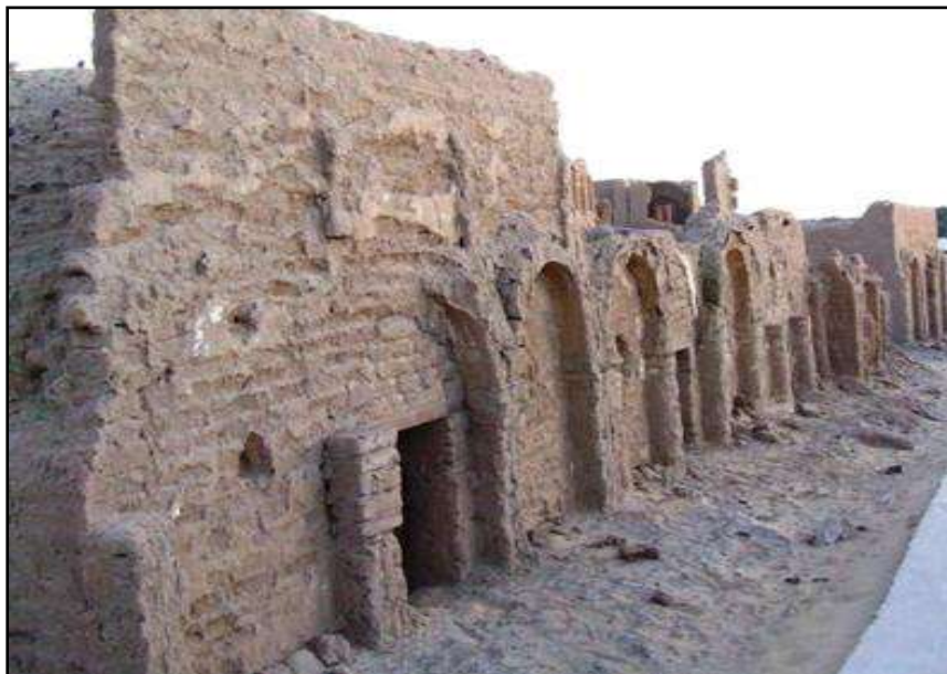
Figure 11. Wind's erosion of tombs façade and weakness of mud bricks
