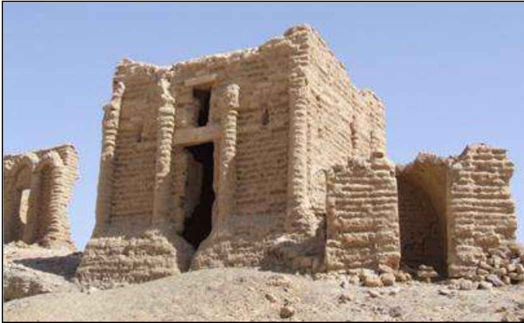
Figure 12. Tombs façade weakness due to wind erosion
