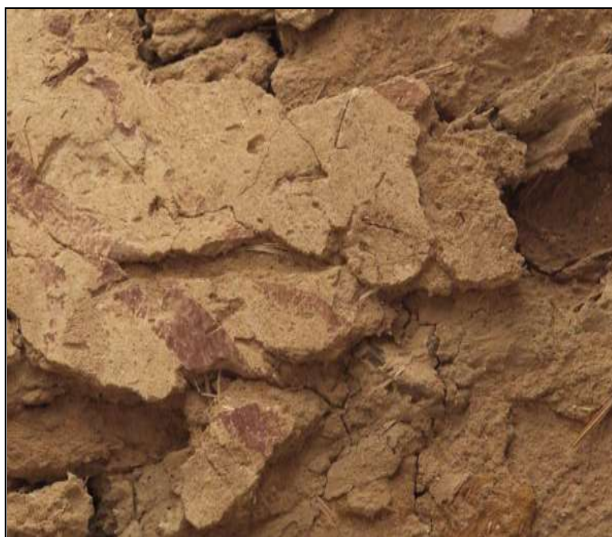
Figure 15. Mud bricks weakness and cracking due to air temperature variation
