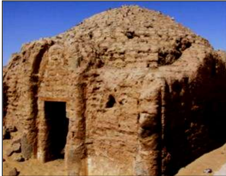
Figure 10. Wind's erosion of mud bricks at El-Bagawat tombs
