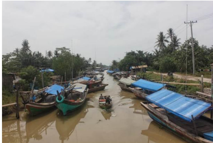
Figure 4. River and Bridge Site
